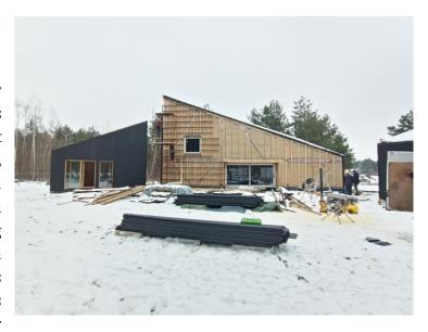
house. Hempcrete, when combined with a timber frame structure, offers significant benefits. It has a negative carbon footprint, helps protect wood from insects, and shields lime from fungi and microorganisms.
